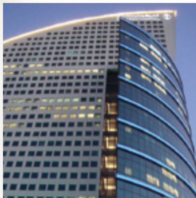
Dubai: Many landmark buildings, including InterContinental Dubai Festival City, feature instant boiling water systems.
