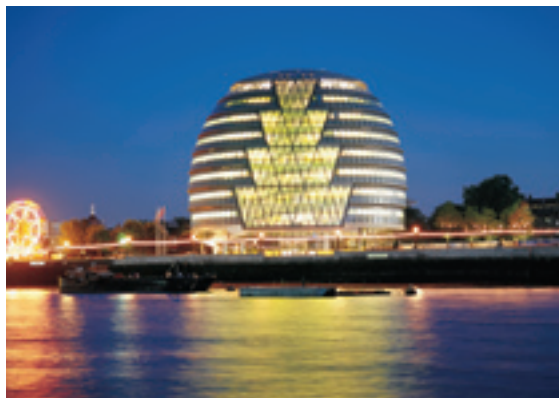
London: offices of The Greater London Authority are also home to instant boiling water systems.
