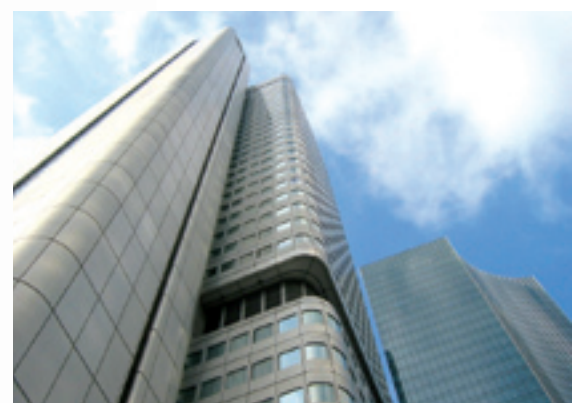
Frankfurt: the head office of the Dresdner Bank is equipped with Hydroboil instant boiling water systems.
